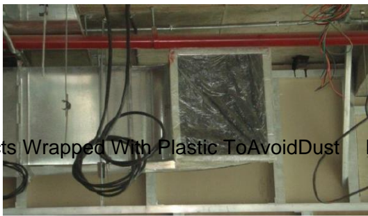
Ducts Stored with Properly Wrapped with Plastic
