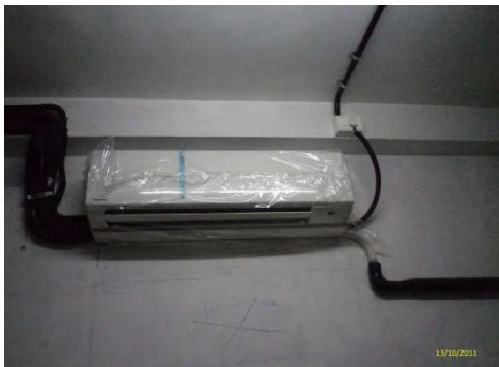
Equipment covered during Construction Phase
